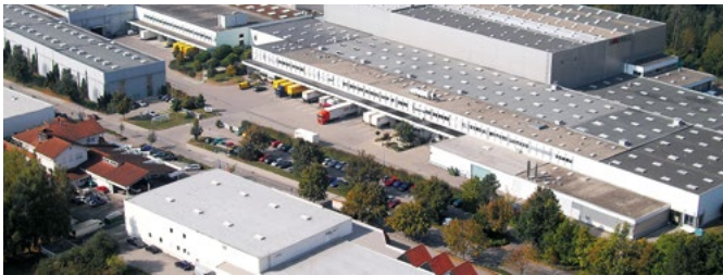
Häfele Distribution Centre Nagold, Germany
