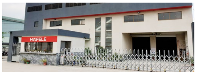
Häfele Production Plant Binh Duong, Vietnam
